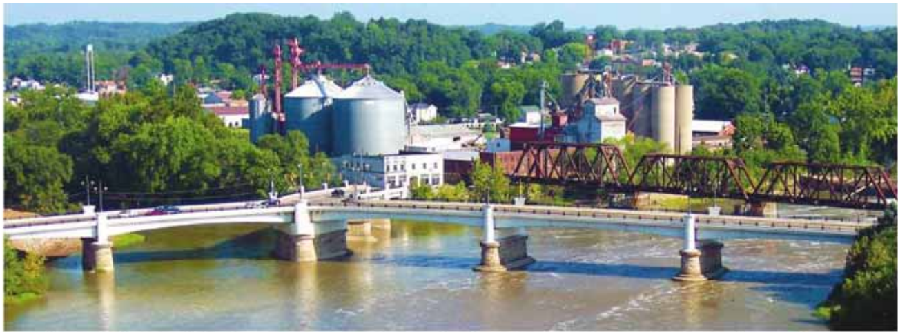
Zanesville: The National Road/U.S. 40 crosses the famous historic landmark, the Y-Bridge, which spans both the Muskingum and Licking rivers.
