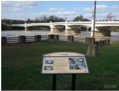
This sign is at the Lock 10 Canal Park. / Submitted photo
