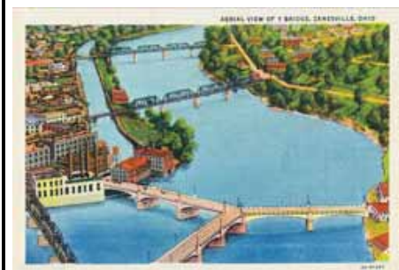
Arial View of Y Bridge, Zanesville Ohio
