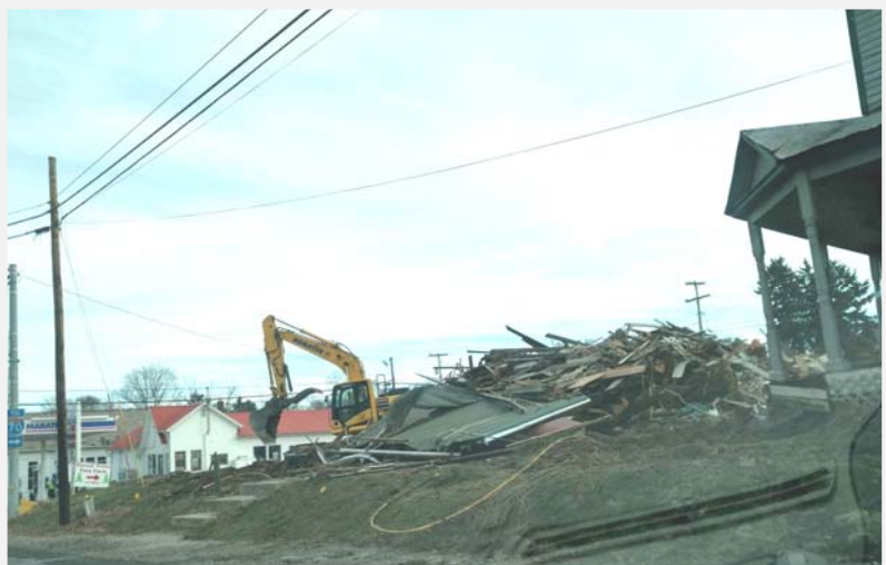
Jacktown Pub Building Demolition. Photo Courtesy of Theresa Clawson Moore
